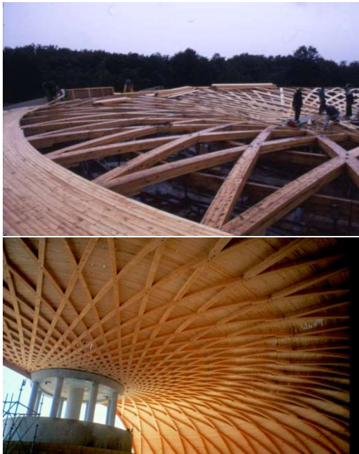
Figure 17: realization, outside and inside
